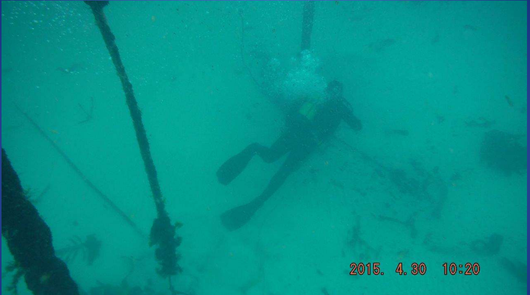
Underwater view of the Shark Repellent Cable in Place at Glencairn Beach (South Africa)
